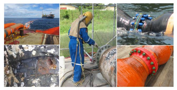
**INCREASE MARINE HOSE SERVICE LIFE BY INCREASING FLANGE CORROSION RESISTANCE** Fit Bolt End Zinc Anodes to greatly increase the corrosion resistance of your marine hose carbon steel flanges. Factory hot dip galvanising and high build epoxy provides good but limited corrosion protection. Operators seeking to extend service life can reduce pitting corrosion by installing Bolt End Zinc Anodes.
